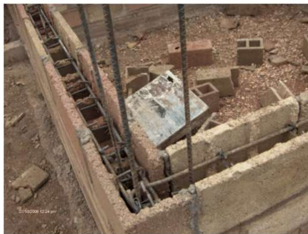
Image 9. Intermediate horizontal reinforcement
