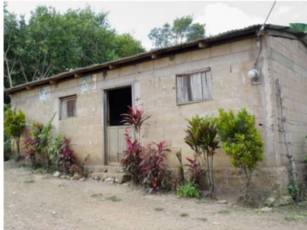
Image 3. Typical house with hollow block walls.
