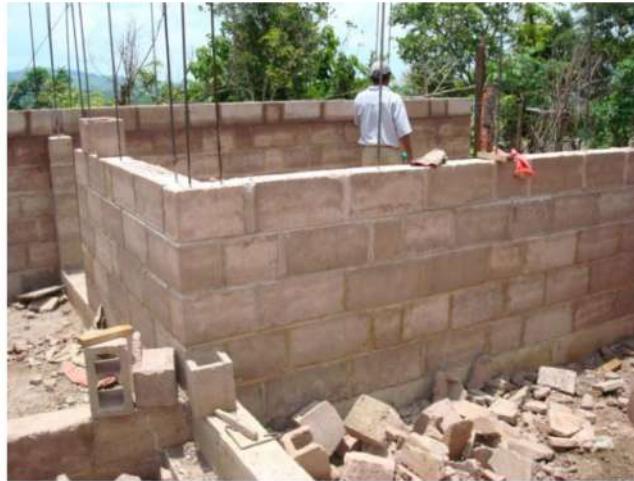
Image 9. Intermediate horizontal reinforcement
