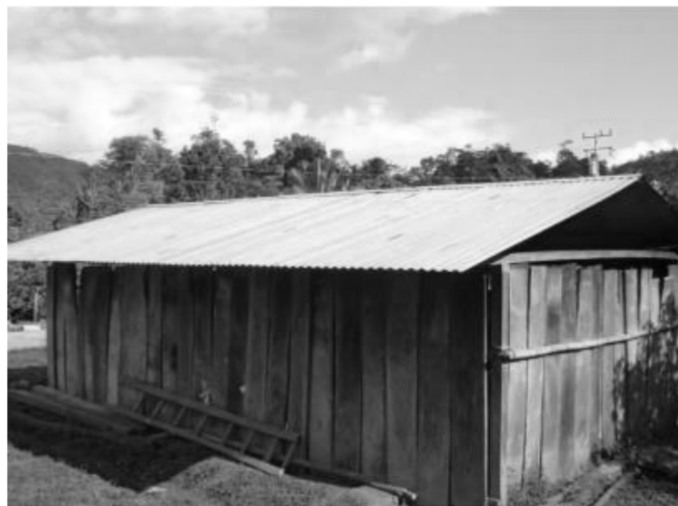
Image 1. Typical rural housing in Yajalón (Chiapas), with wooden walls and a sheet roof.
