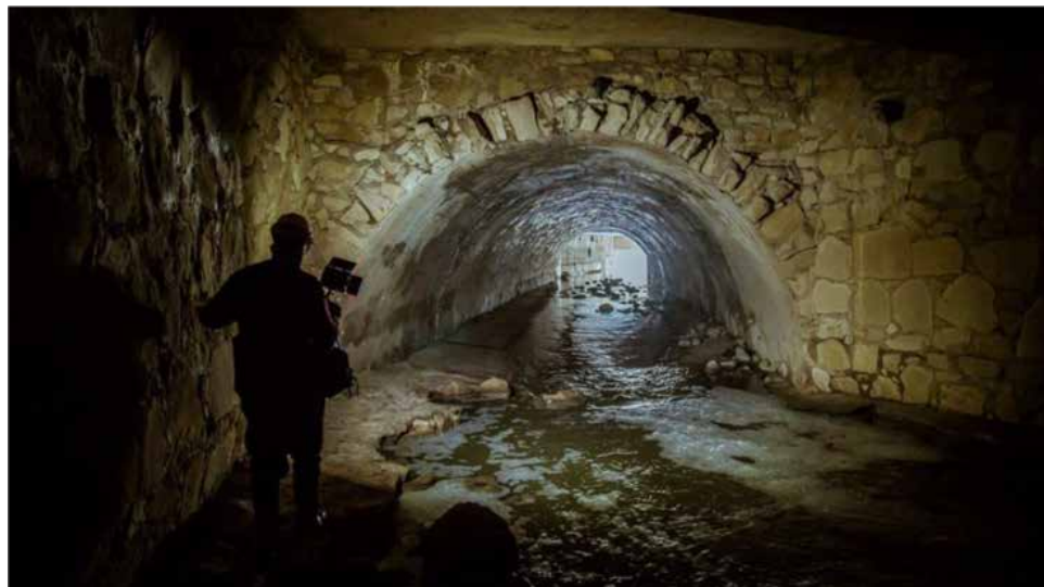
Figure 9. General view section of the stone underground culverts-arch's (Tavera, 2018)
