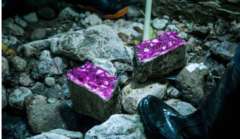
Figure 11. In-situ carbonation front measurement in a concrete sample of the slab, using an acid-base indicator solution: phenolphthalein (Tavera, 2018)
