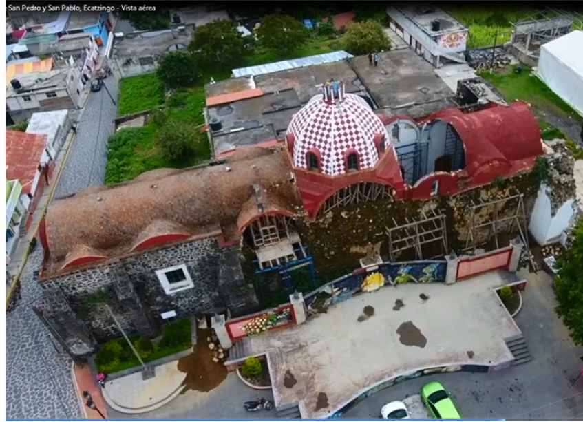
Figure 4. Vault with lunettes. Source: Elaboration INAH (2018)
