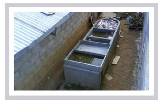
**Tank with laminated siphon (TLS).** The TLS is a hydraulic structure (tank) used to supply water intermittently to agricultural parcels (up to one hectare) small home gardens. This system has a discharge tube in the shape of a laminated siphon, which can save large amounts of water (up to 50 out of every 100 liters used) compared to continuous surface irrigation. The fundamental equation governing its intermittency for a constant flow input is:
