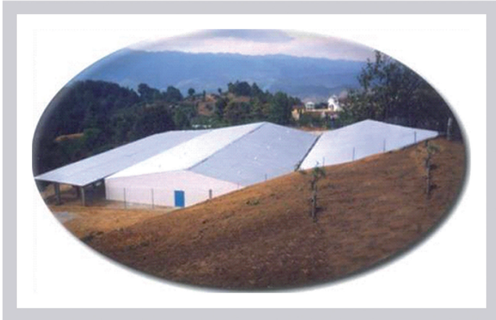
Photo 1. Collector rainwater, Yalentay, Zinacantán, Chiapas.
