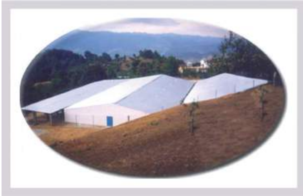
Photo 1. Collector rainwater, Yalentay, Zinacantán, Chiapas.
