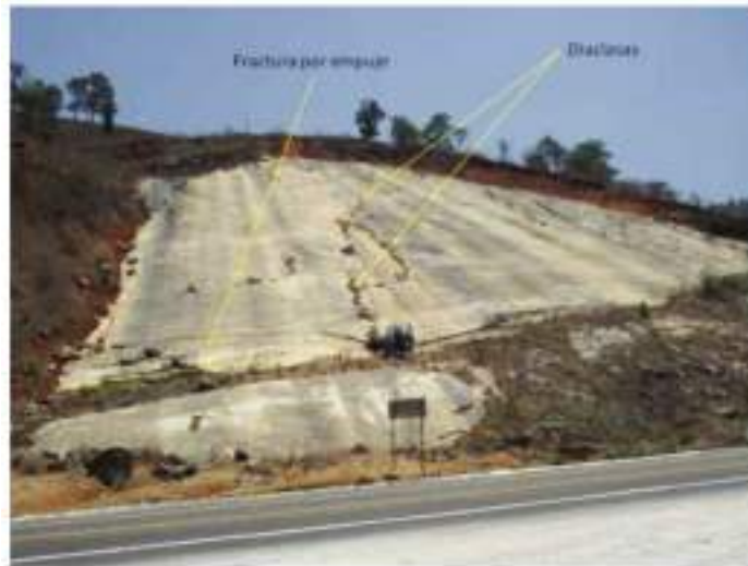
Photo 2. Tuxtla Gutiérrez-San Cristóbal Highway. Paz, 2013
