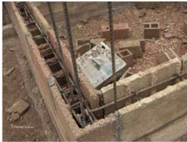
Image 9. Intermediate horizontal reinforcement
