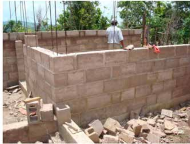
Image 9. Intermediate horizontal reinforcement
