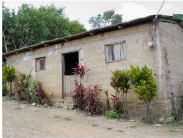
Image 3. Typical house with hollow block walls.
