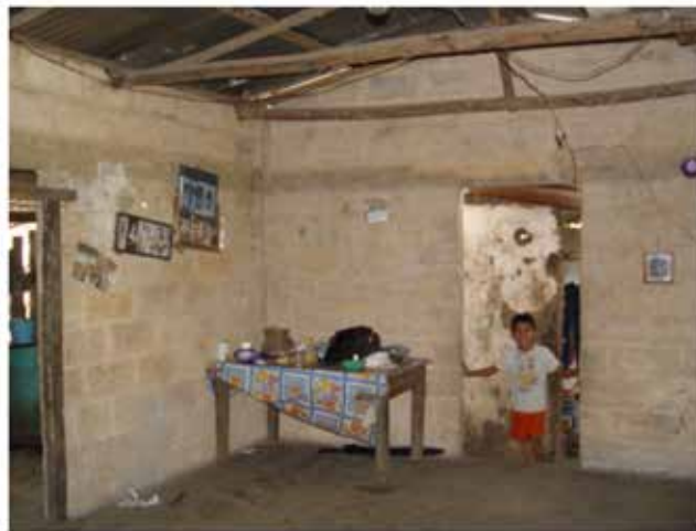
Image 2. Inside of a hollow block house
