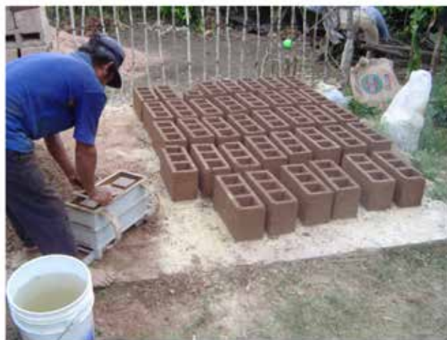
Image 6. Hollow block pieces with three cells
