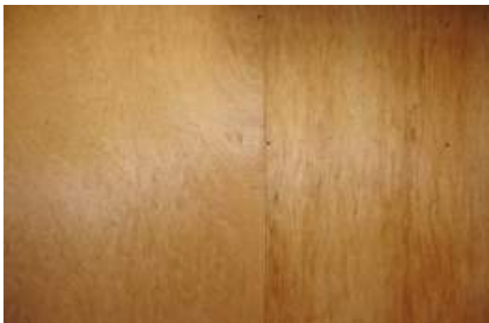
Image 4. Wall finished and lined with plywood, to cover the lead sheets
