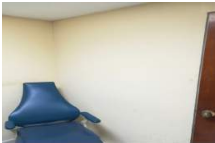
Image 1. Walls without the lead lining
