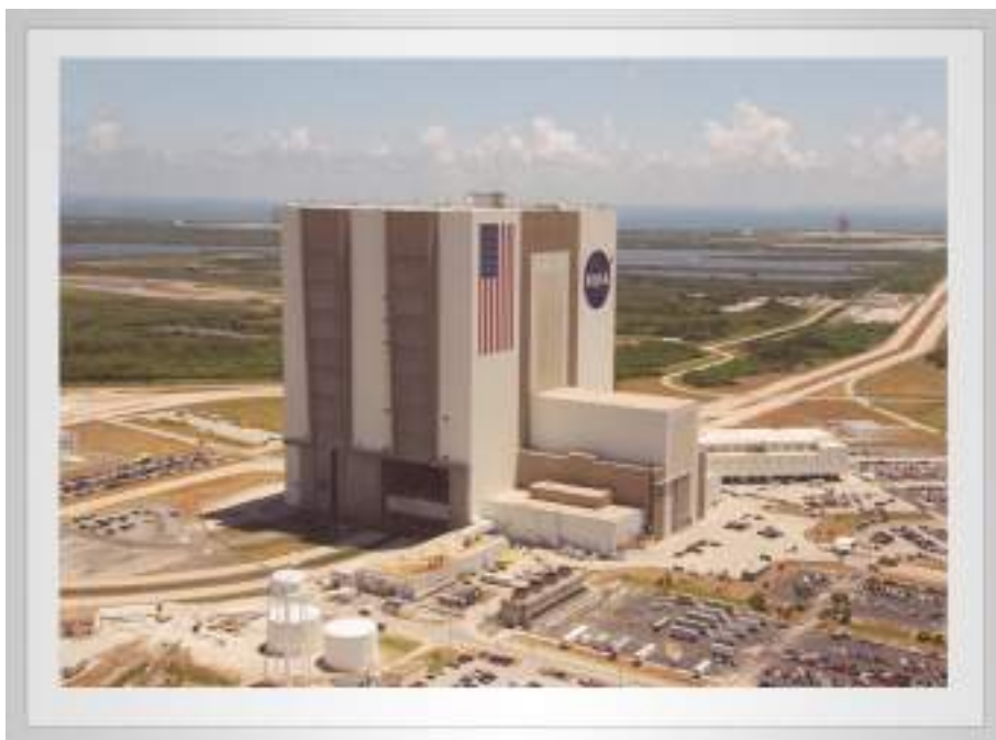
Figure 4. The Vehicle Assembly Building (VAB) was built for the Apollo program (1964). The VAB was designed to store and assemble the 110 meter tall Saturn V rocket. One of the most notable characteristics of the VAB is its 139 meter tall doors (they are the tallest doors in the world). The VAB is also used to mount the NASA Space Shuttle. The VAB is used for the mounting and assembly of the SLS and the MPCV. Photo courtesy of NASA.
