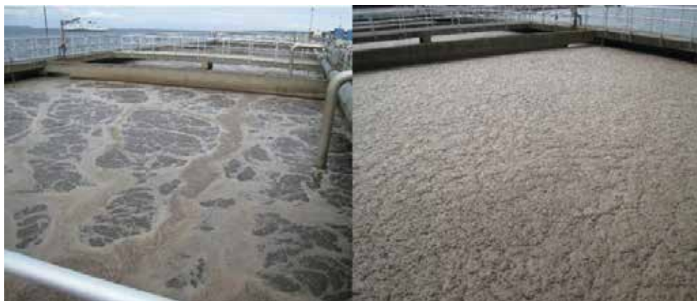
Figure 2. Example of foaming in a conventional biological treatment system
