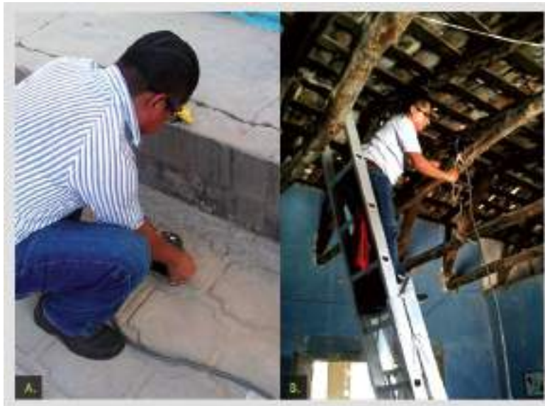
Figure 2. a)Installing the accelerometer on the floor, b) Installing the accelerometer inside the house
