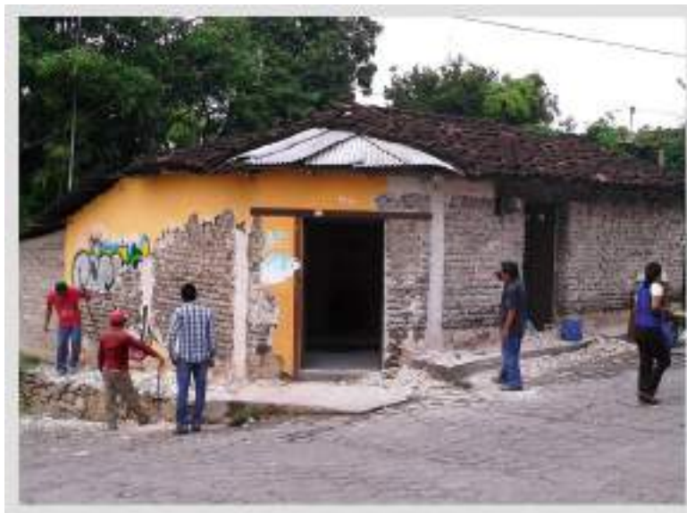
Figura 4. Removal of the existing mortar on the house
