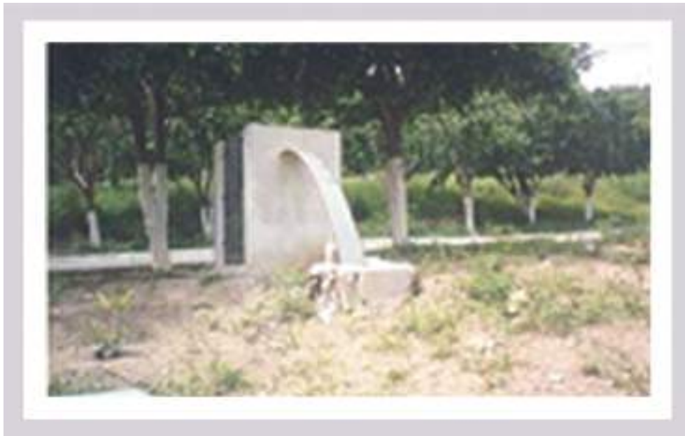
Photo 10. Laminate siphon tank
